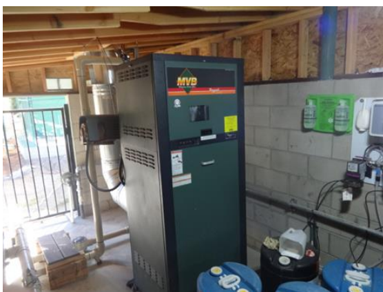
Description: Swing Barriers
